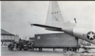
One of the 14 portable "slide" used in transporting the PM-1 to Sundance.
